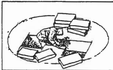
Cutting blocks for a snowhouse, the builder stands inside the circle that outlines the dwelling to be constructed.
